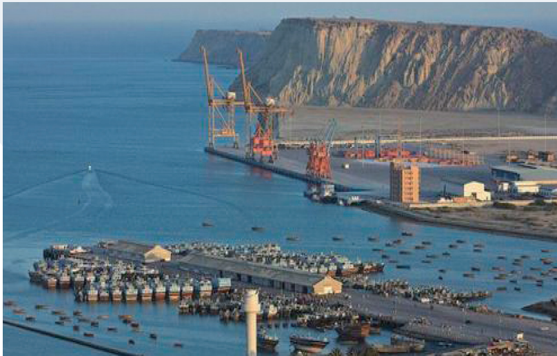
Picture 7: The Gwadar Port project (Phase I) built with the Chinese aid is located in Gwadar Town, Balochistan, Pakistan. The project includes building three multi-purpose berths at the 20,000 tonne scale, and the structure is designed to berth container ships with 50,000 tonne scale. The construction commenced in 2002 and completed in 2008. (Picture from the Internet)
