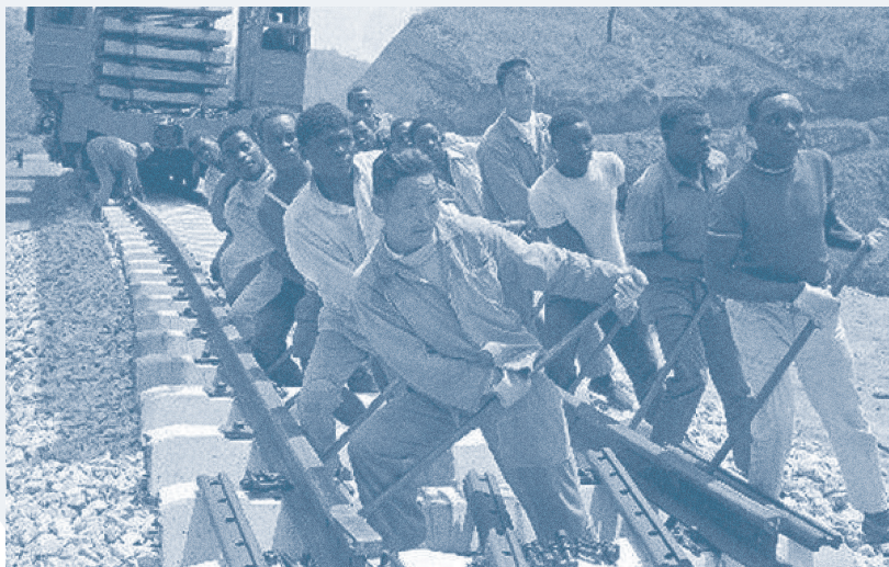
Figure 2: Chinese and foreign engineers and technicians are laying railway tracks during the construction of the TAZARA Railway. (Picture from the Internet)
